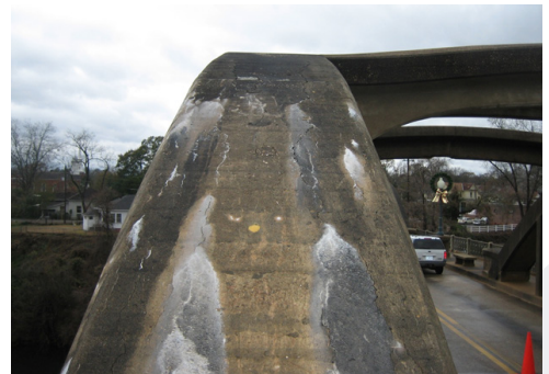
Figure 2. ASR-affected Bibb Graves Bridge in Wetumpka, Alabama, showing cracking and gel exudation features.
