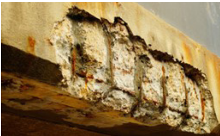
Corrosion damage on a concrete bridge on a busy thoroughfare in Frankfurt, aged about 50 years.
